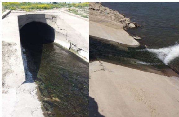
Slika 8. Izlaz pročišćene otpadne vode iz kanala u recipijent, rijeku Savu Fig. 8. Exit of purified wastewater from the canal to the recipient, the Sava river
