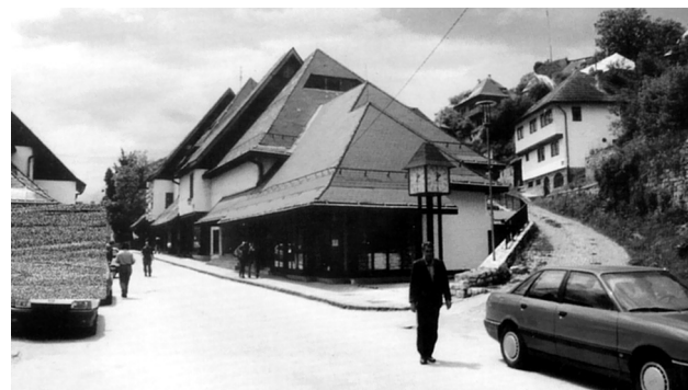
Figure 6 Shopping center "Jajce" built during 1976. Slika 6. Robna kuća "Jajce" izgrađena 1976.
