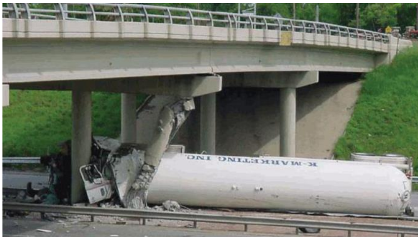
Figure 1 Impact between vehicle and column (U.S. highway) [8]
