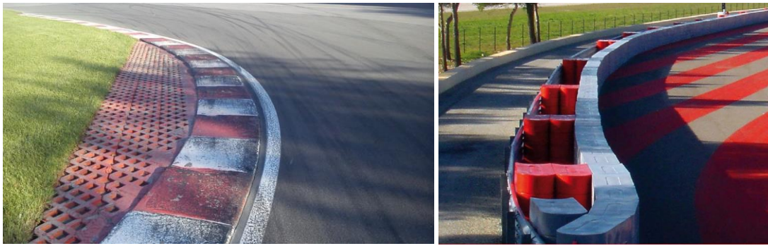
Figure 6 Inner curbs and TECPRO energy dissipation system [16, 17]
