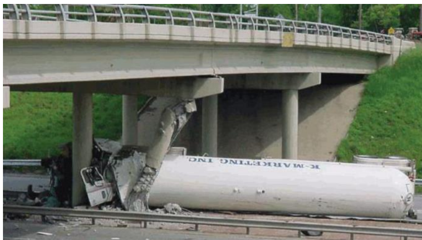
Figure 1 Impact between vehicle and column (U.S. highway) [8]
