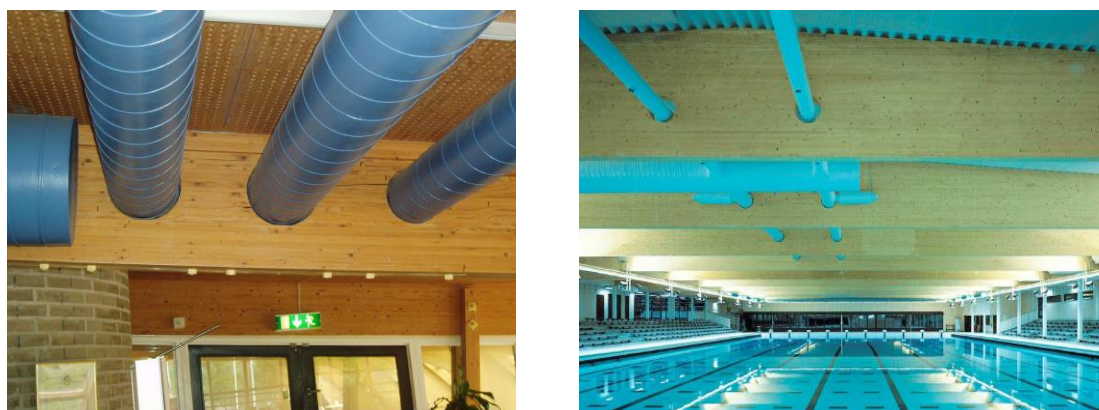
Figure 1 Glulam beams with openings [1]
