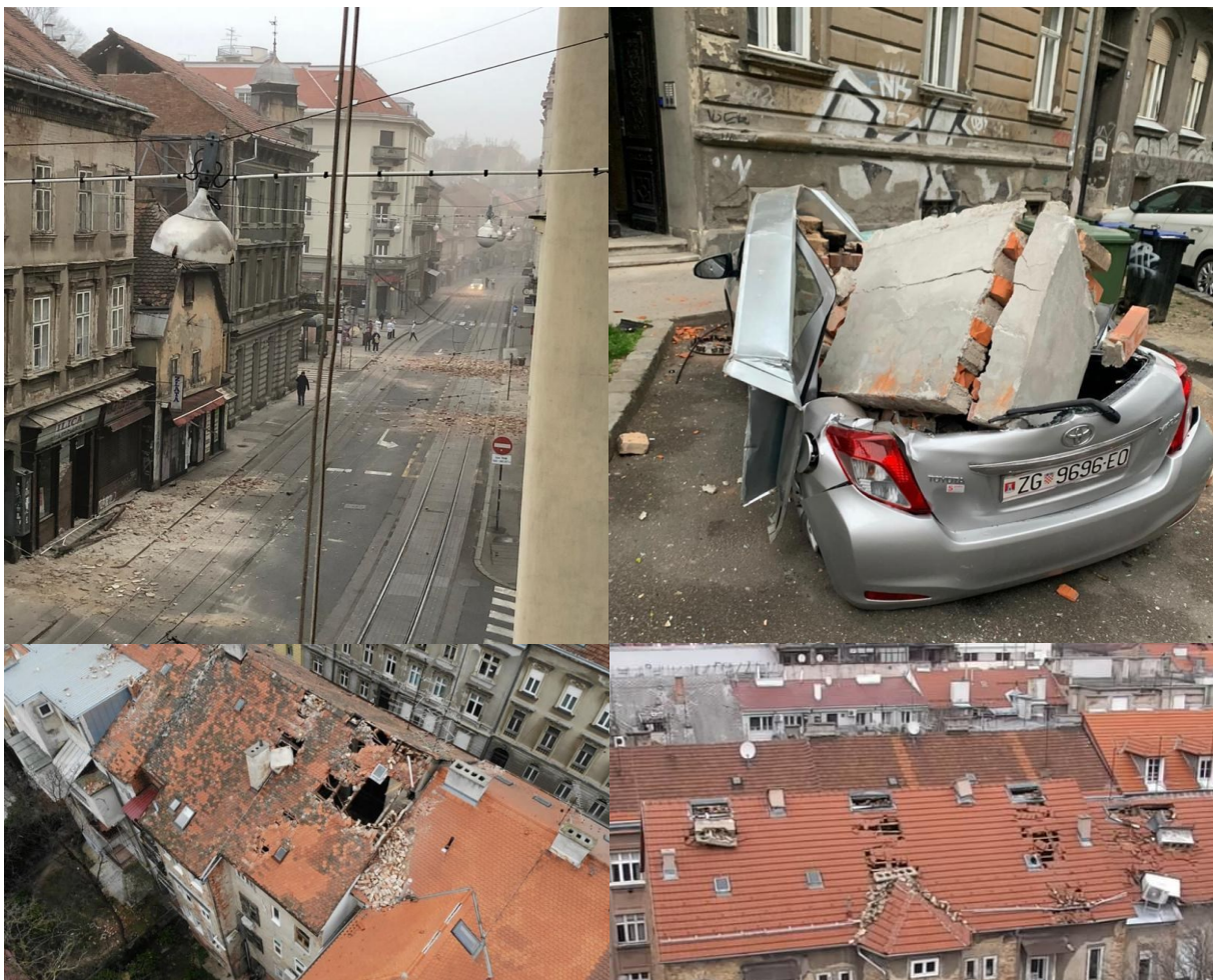
Figure 5. Damage in Zagreb after 22 March M5.5 earthquake. Noticeable roof tile loss and chimney collapse
