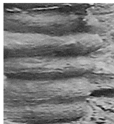
Figure 10 Ground after jet grouting Slika 10. Tlo injektirano mlaznim postupkom
