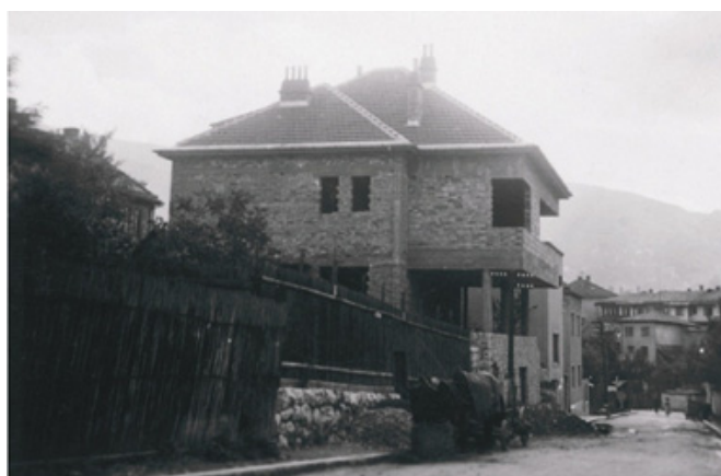
Figure 3. Kopčić House constructed on Safvet-beg Bašagić Street in 1939 [15].
