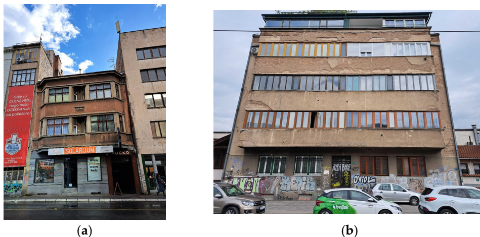
Figure 1. (a) Damić House (author’s source); (b) Jakub-Paša Building, Obala Kulina bana Street (author’s source).
