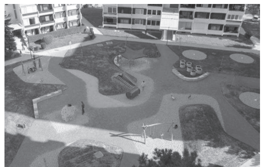
Figure 10 The Pilot Action Target Area After Renovation
