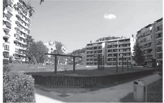
Figure 9 The Pilot Action Target Area Before Renovation
